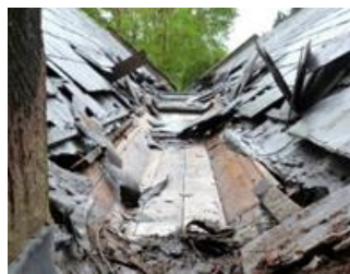
Metal Theft, St Peter's Church, Plemstall (Chester and Cheshire West Council)
